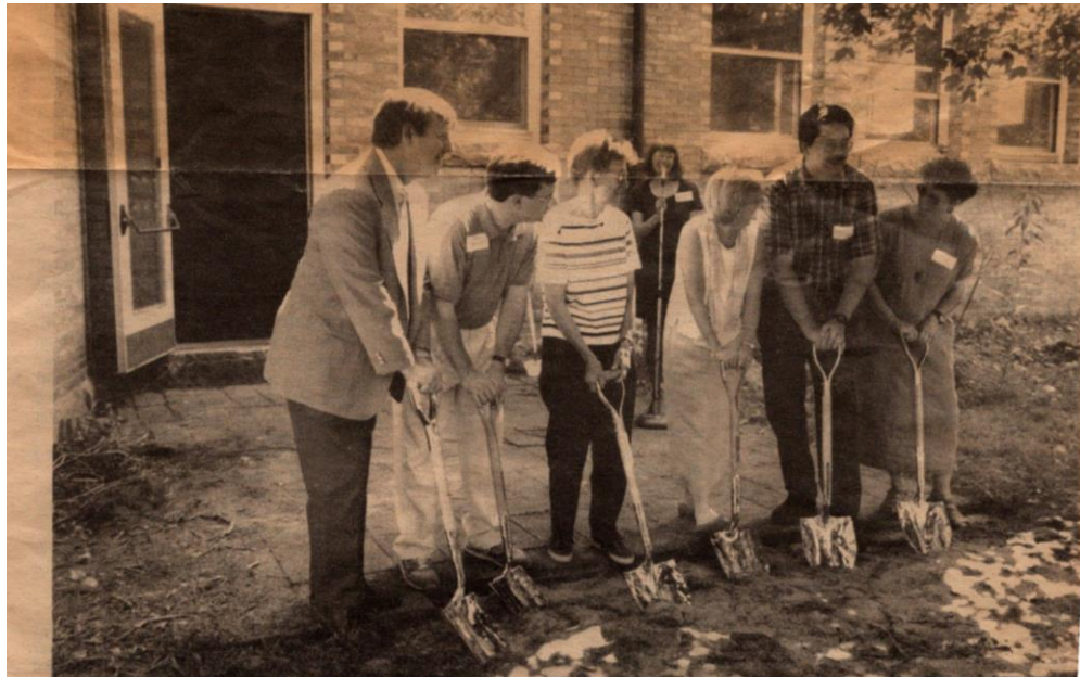
Digging in! The Public Library held its ground breaking ceremonies last Saturday with officials using shiny shovels to make the symbolic first cut into the area where the library expansion will be constructed. Shown in photo are Frank Adams, Stahl Assoc. Architects, (left to right); Ed McNierney, Building Committee member; Katie Madigan, Library Trustee; Owen S. Shuman, Library Director; Mike Muse, Castagna Construction Corp.; Martha McLure, co-chair Library Endowment Committee. Valerie Jenkins, Library Trustee, is in the back.
